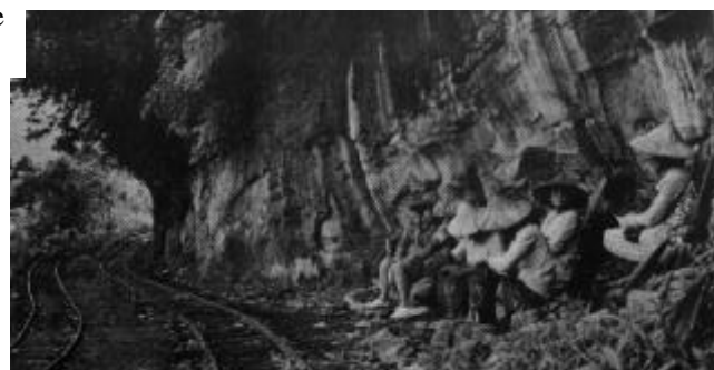
fig. 8 – The helper station. All coal trains pick-up a helper here for the steep grade to the north portal
