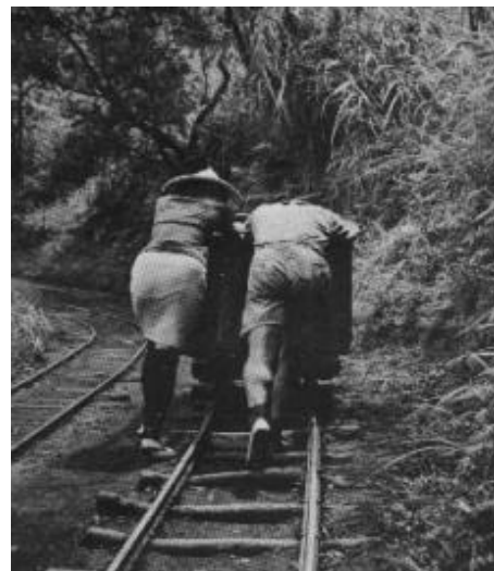
fig. 7 – The earth between the ties has been pounded down by the pressure of the pusher’s feet.
