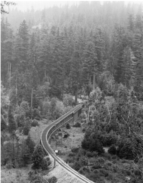
South Pacific Coast Railroad Trestle at Big Trees.
