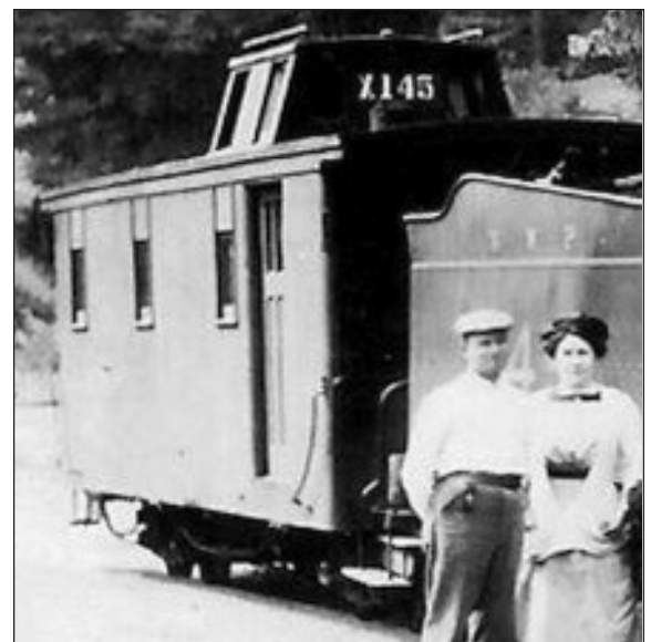
NWP caboose 6101 (detail of larger image) at Monte Rio, CA circa 1911-12. Note the train number or "marker" units in the cupola's center window, and one of two small oil lamp vents in the cupola roof. [NWPRRH Archives]
