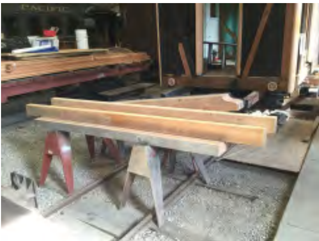
Photos: New needle beams cut by Bill Wissel
