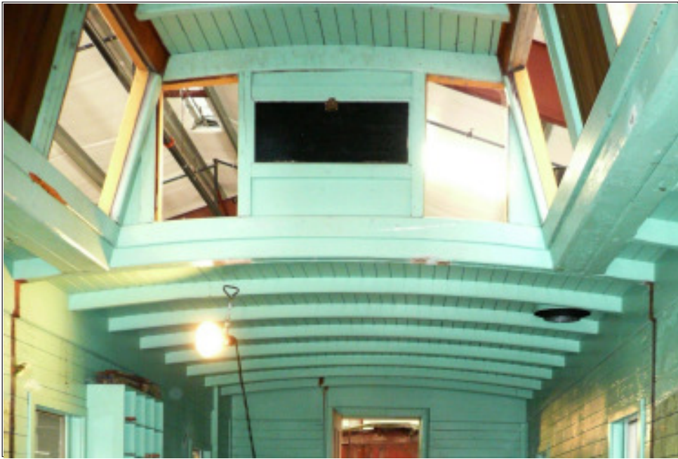
Inside of Bethlehem rebuilt cupola - Kevin Bunker photo
