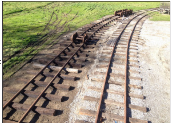
New spur track.
