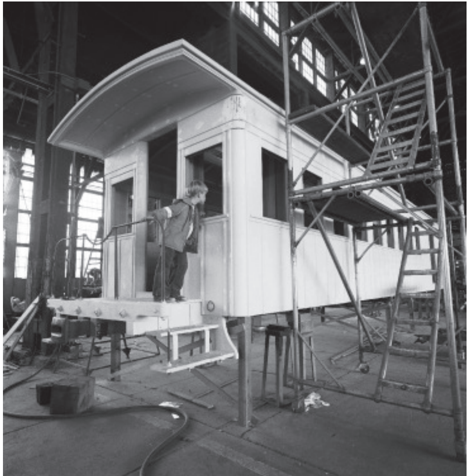
The tired-out accumulations of Nevada Central Railroad alterations and finishes have given way to a 1970s reversal staged inside CSRM's first restoration shop at Sacramento. A young Haig MacGregor (son of our Collections Manager) gives the nearly complete “Monterey Car” a visual inspection. With primer already done and sanded smooth, painters will next apply the first layers of a pale yellow body color, while across the way, other craftsmen are rebuilding the combine's trucks to like-new condition.
