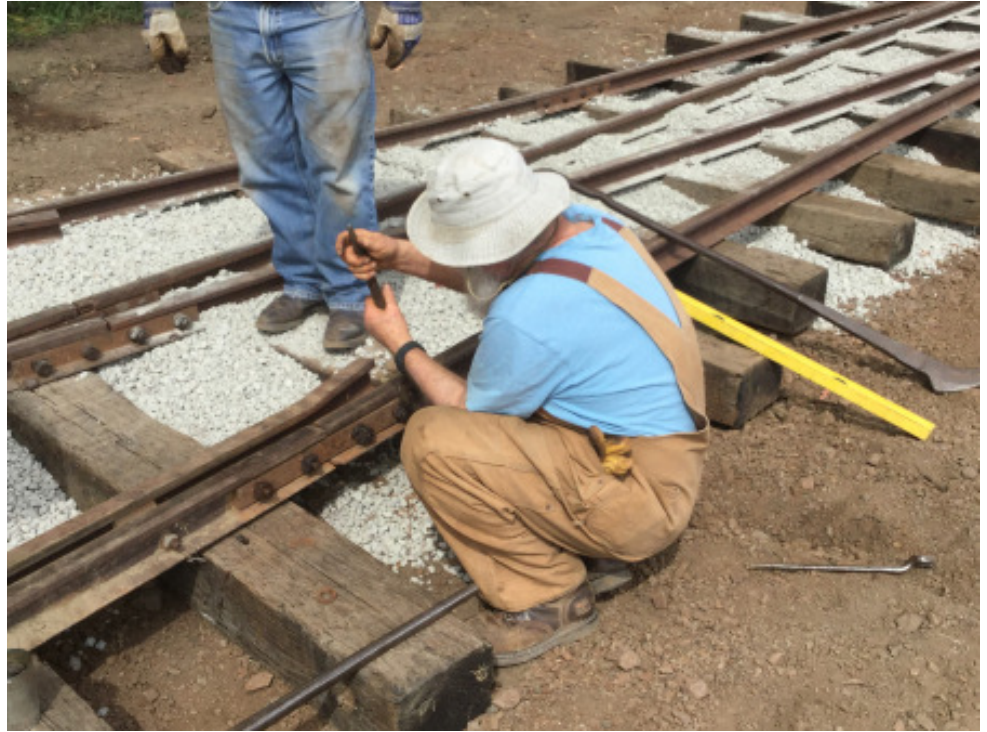
Gene Arrillaga bolting a joint bar. Photo by Jack Burgess
