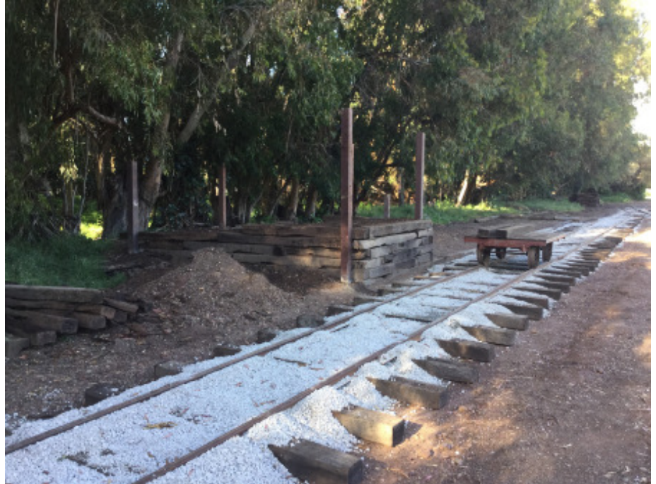
Track all finished and ballasted. Photo by Jack Burgess
