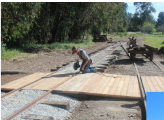
David Waterman finished up Deer Park's new walkway. Photo: Barry Lependorf
