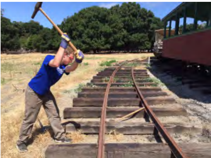
Bobby Goldie spikes rail on track 5
