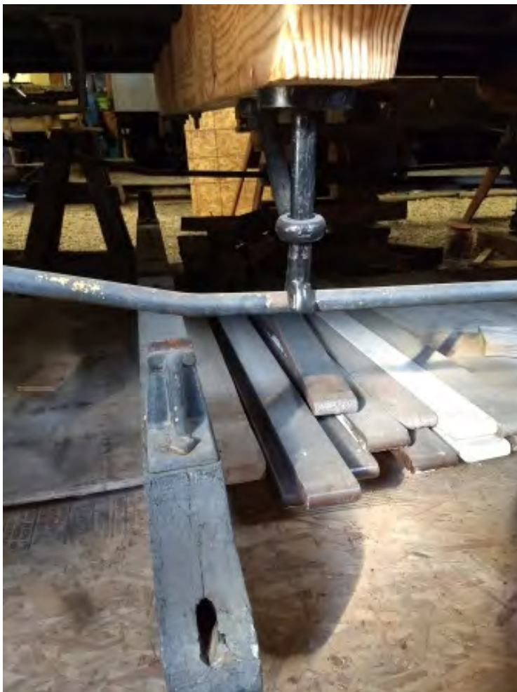
Illustration 6: The 'new' Queen posts (top) compared to the old (upsides down on bottom)
