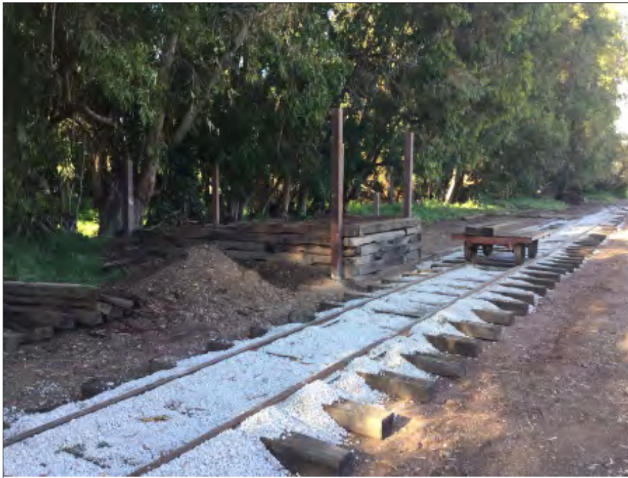
Track all finished and ballasted. Photo: Jack Burgess
