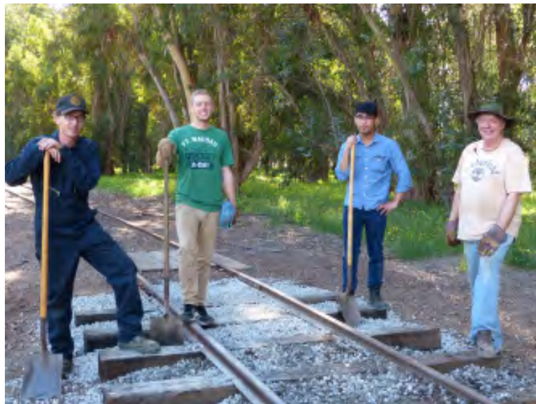
Left to right: Bobby Goldie, John Goldie, Jay Martinez and David Waterman tamp and adjust ballast at Deer Park.
