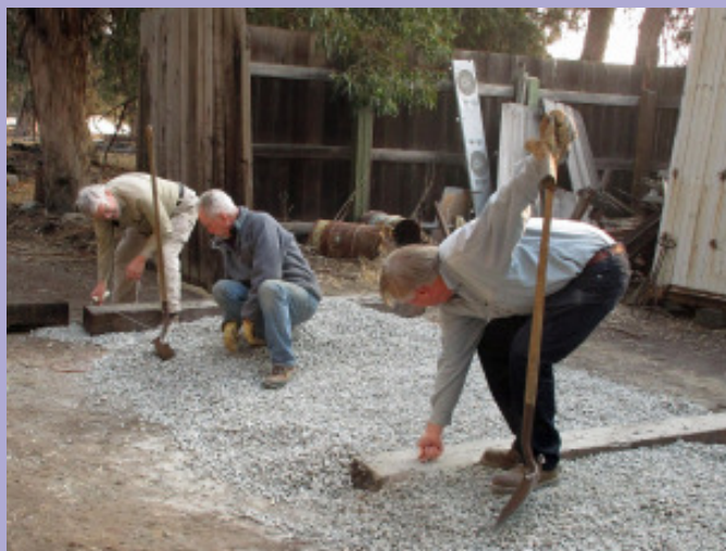
John Stutz, Jack Burgess, and John Goldie (left to right) prepare the base for the new event container. Photo by Don Marenzi
