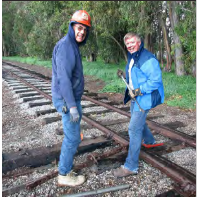
Steve Rusconi (on left) with Track Manager John Goldie working on the new switch at Deer Park. Photo: Don Marenzi
