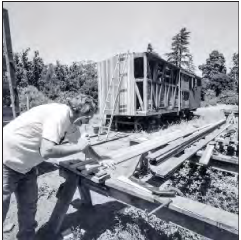
Rich Neelson works on restoring box car 472. Photo: Bruce MacGregor
