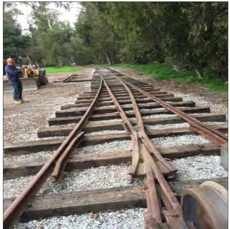
Steve Rusconi watches push car go through new switch at Deer Park.
