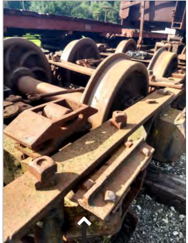
Truck with cut down rail repair.
