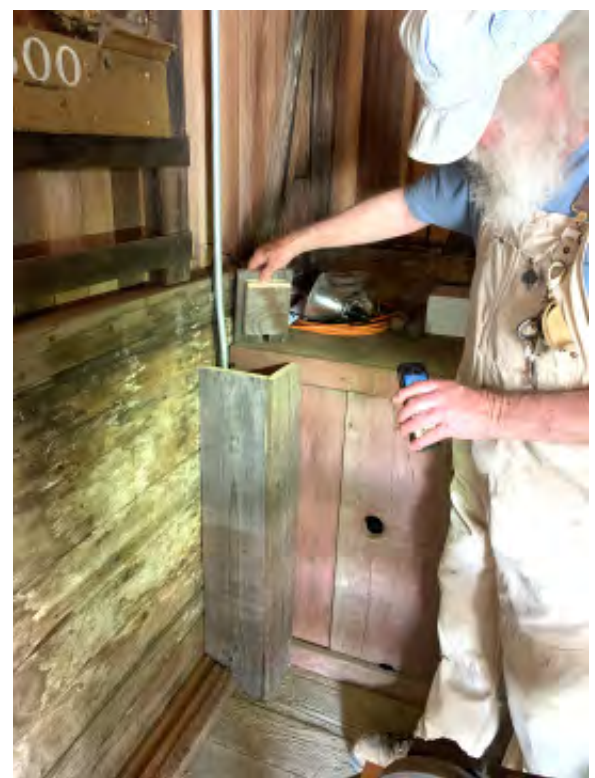
Gene Arrillaga shows the wooden box & cover made by Tony Peters to hide the electrical cable for the new lights in the museum car. Photo: J. Burgess
