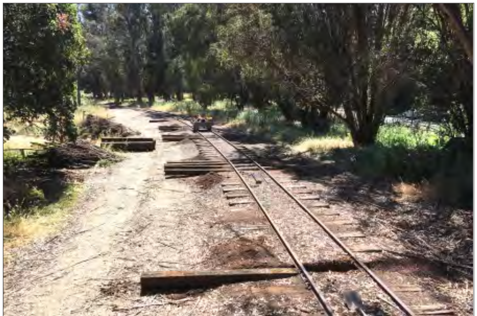
John Goldie and David Waterman replaced 12 ties in one day! Photo: David Waterman
