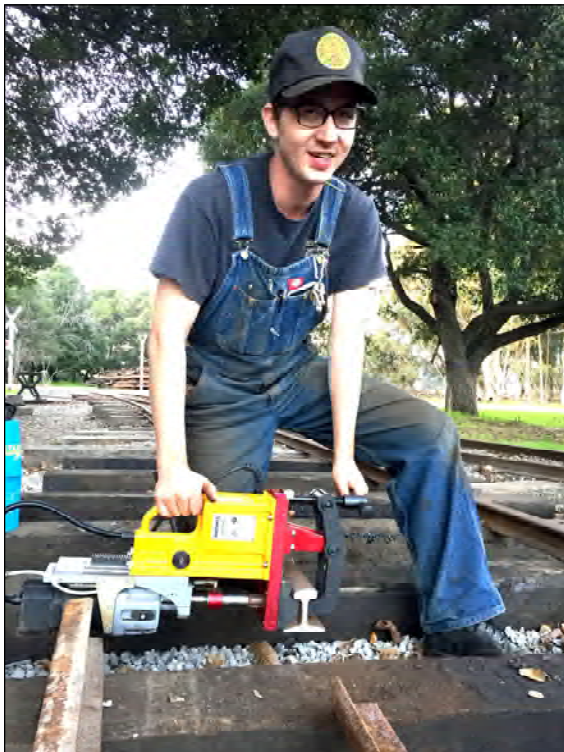
David put the new electric rail drill to work right away
