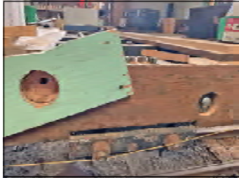
A router was used to counter-sink the bolts. That will create a smooth surface when the siding goes on.
