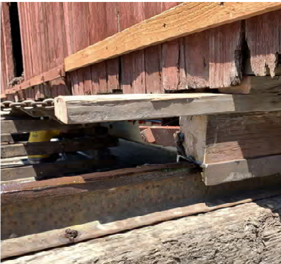
Box car on skid blocks to slide the car on the rail over to the cribbing. Photo: Editor
