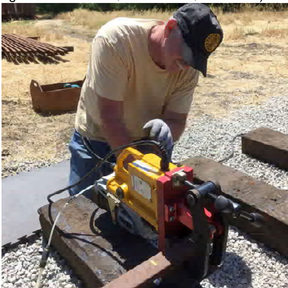
Barry Lependorf drilling bolt holes in rail. Photo: David Waterman.
