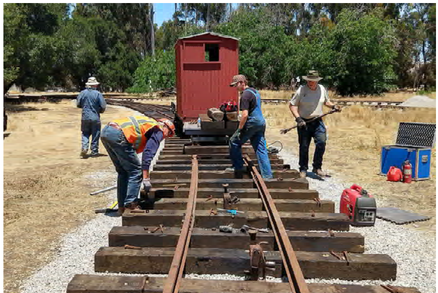
MOW crew measures rail location on ties & checks the gauge (left to right: Bruce Sorel, Steve Rusconi, David Waterman, John Goldie).
