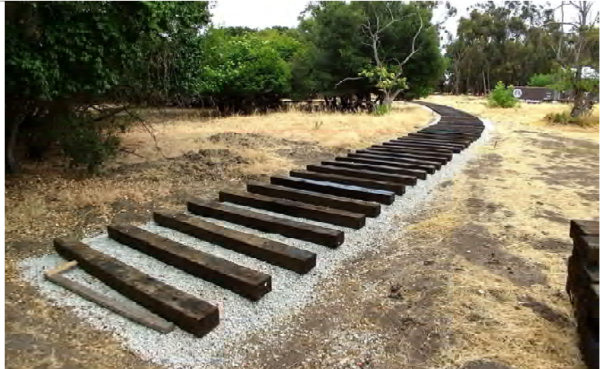
Track crew laid out ties for the first section of the loop leaving the Car Barn area.
