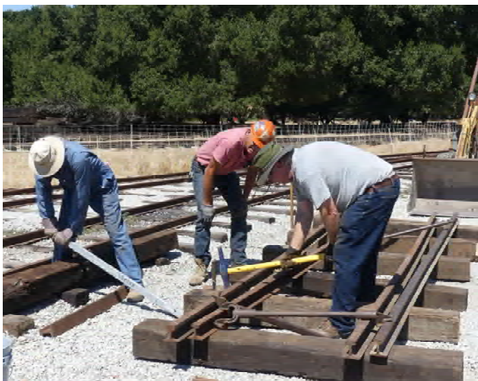
John Goldie drives a spike into the new snap track while Bruce Sorel pinches the tie up. The guys took turns on this hot day. Photo: JS Burgess
