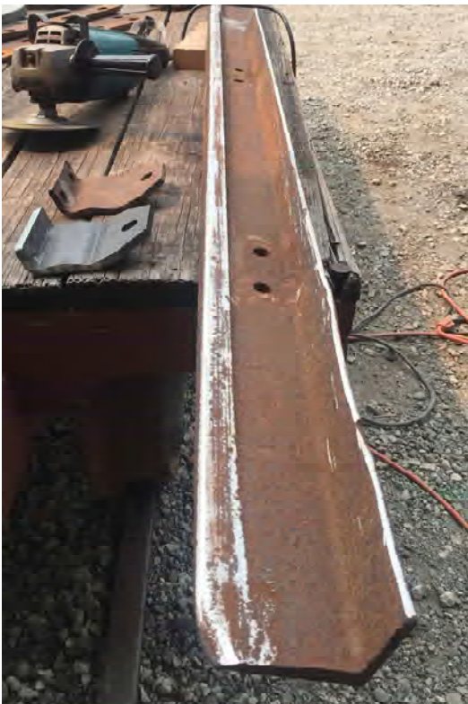
Point repair in progress. Grinding, welding and flat bar installed. Note the transit plates on the table... Steve fabricated a new transit plate to match the other one (he donated both).
