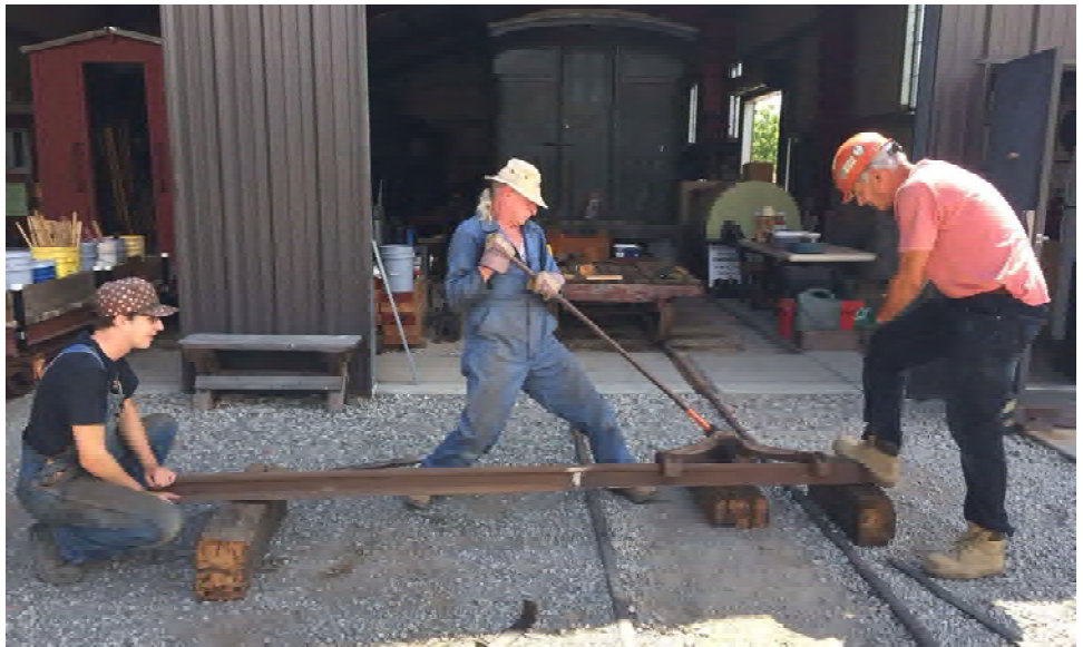
Bruce Sorel (center) bends the point rail straight with the Aldon Rail Bender while David Waterman (left) and Steve Rusconi (right) steady it. Photo: John Goldie
