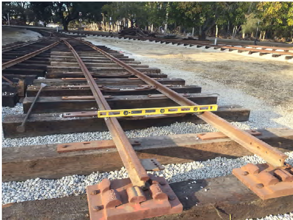
The level swing rails of the future stub switch.
