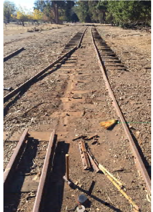
Removal of two worn pieces of rail on the right-of-way.
