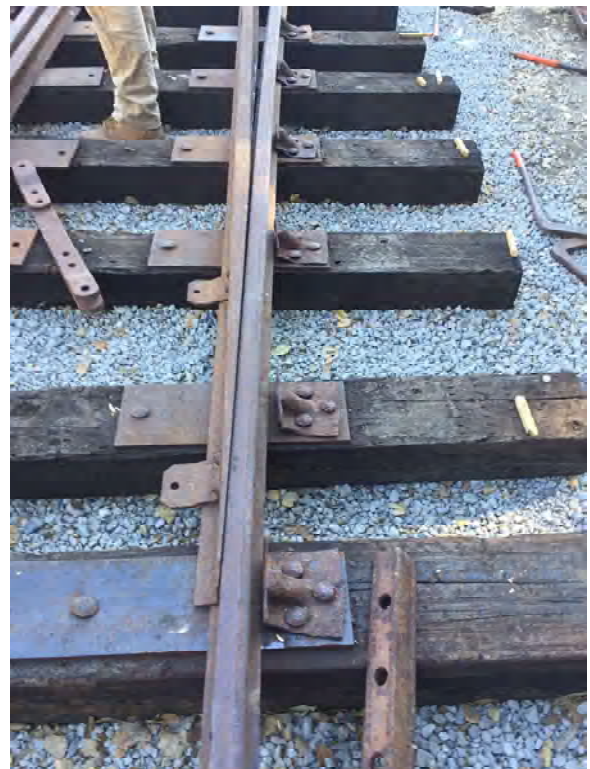
Here is the nested point for a turnout after adjustments were made for a good fit.
