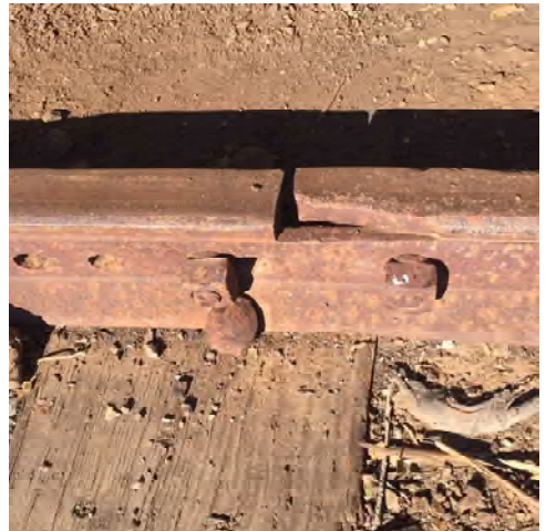
Track defects: missing bolt, broken rail and broken washers.
