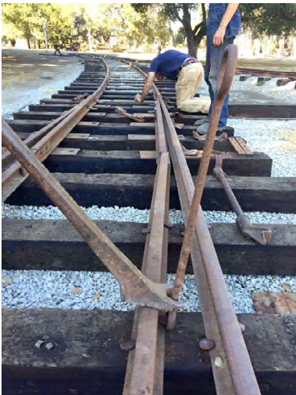
When we can't get the claw foot spike puller to fit in, we use the Roadmaster spike puller. It grabs the head of the spike. The 4 knobs up the shaft are pull points for the claw spike puller.
