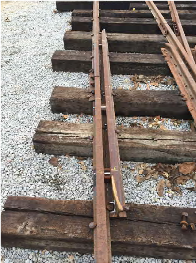
Installed guard rail.
