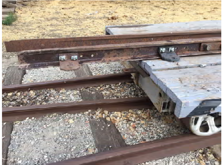
The points are on the push car for some final cleanup work. The transit clip is now in the correct location.
