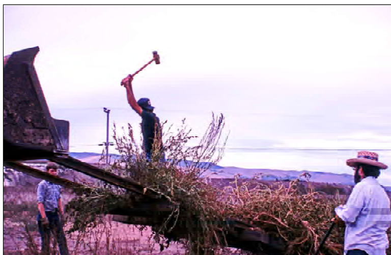
It worked much better to lift the rail then hammer the ties off. Volunteers: Bill Barbour, Rich Neilson, Bruce MacGregor (left to right)
