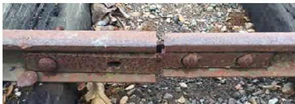
Image 2: SPCRR custom-built compromise joint. Note the gauge side and head alignment.
