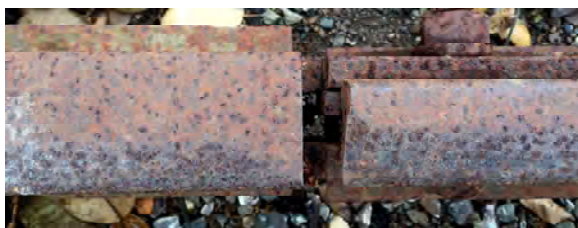
Image 3: Top down view showing the double bar on the 25# rail to align the gauge side.
