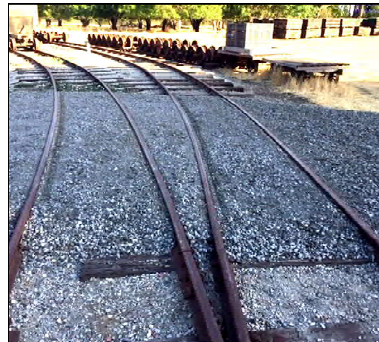
The new tractor crossing of tracks 4 and 5-placement to beyond the clear post to not block any storage tracks., Photo - John Goldie
