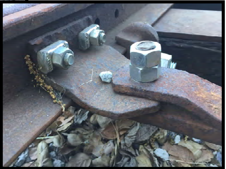
Figure 2 - #1 Switch Rod with nuts up on the bolt.
