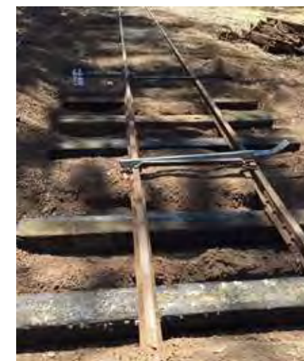
7/10/21: Next is the new ties inserted and the phantom turnout removed.
