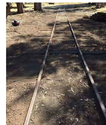
Last step - the cleaned up track is swept and gauged. Ready for operation.
