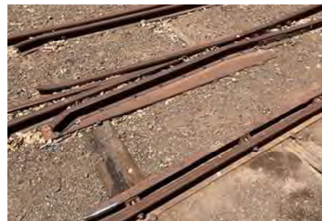
New guard rail installed to protect non-diverging moves on track 1 at Ardenwood station, 6/13/21. Photo: John Goldie
