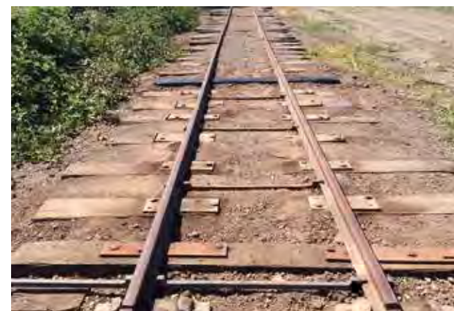
Swing rail section with new #1 tie and also lead tie, 6/20/21.
