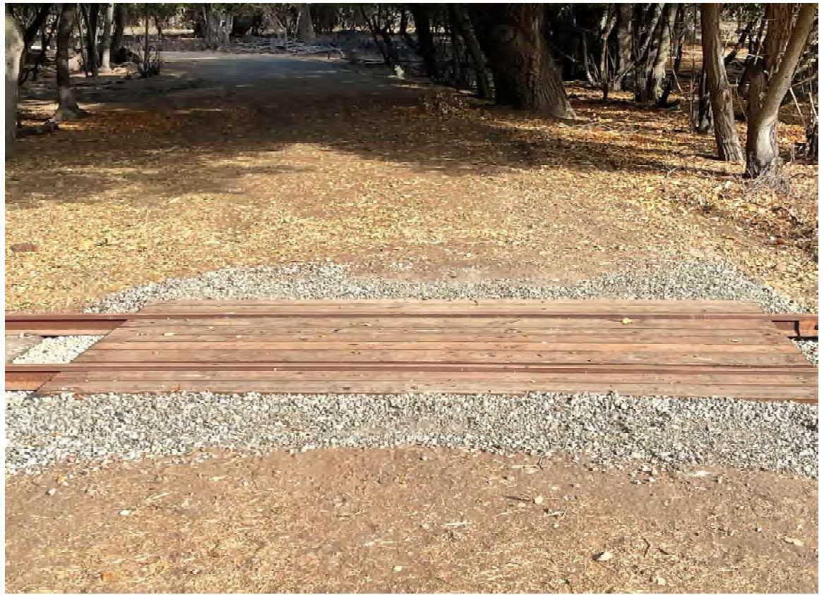
Once we received approval for the track extension/loop from EBRPD, the track crew installed the first crossing at the William Patterson road, then started laying track headed west. The wood crossings offer a solid flat crossing with less maintenance than a gravel crossing. Photo: JS Burgess
