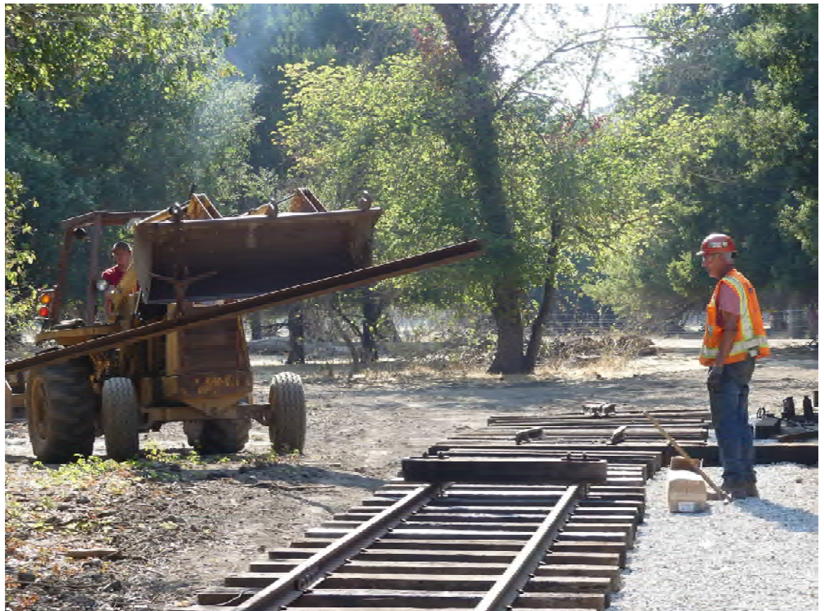
This photo was taken last weekend. You can see they have made it to the trees shown in the distance in the previous photo. Bobby Goldie on the tractor moves the next piece of rail as Steve Rusconi directs him where to place it. A plastic tarp was placed under the ballast as this area was prone to poison oak sprouts. Photo: JS Burgess
