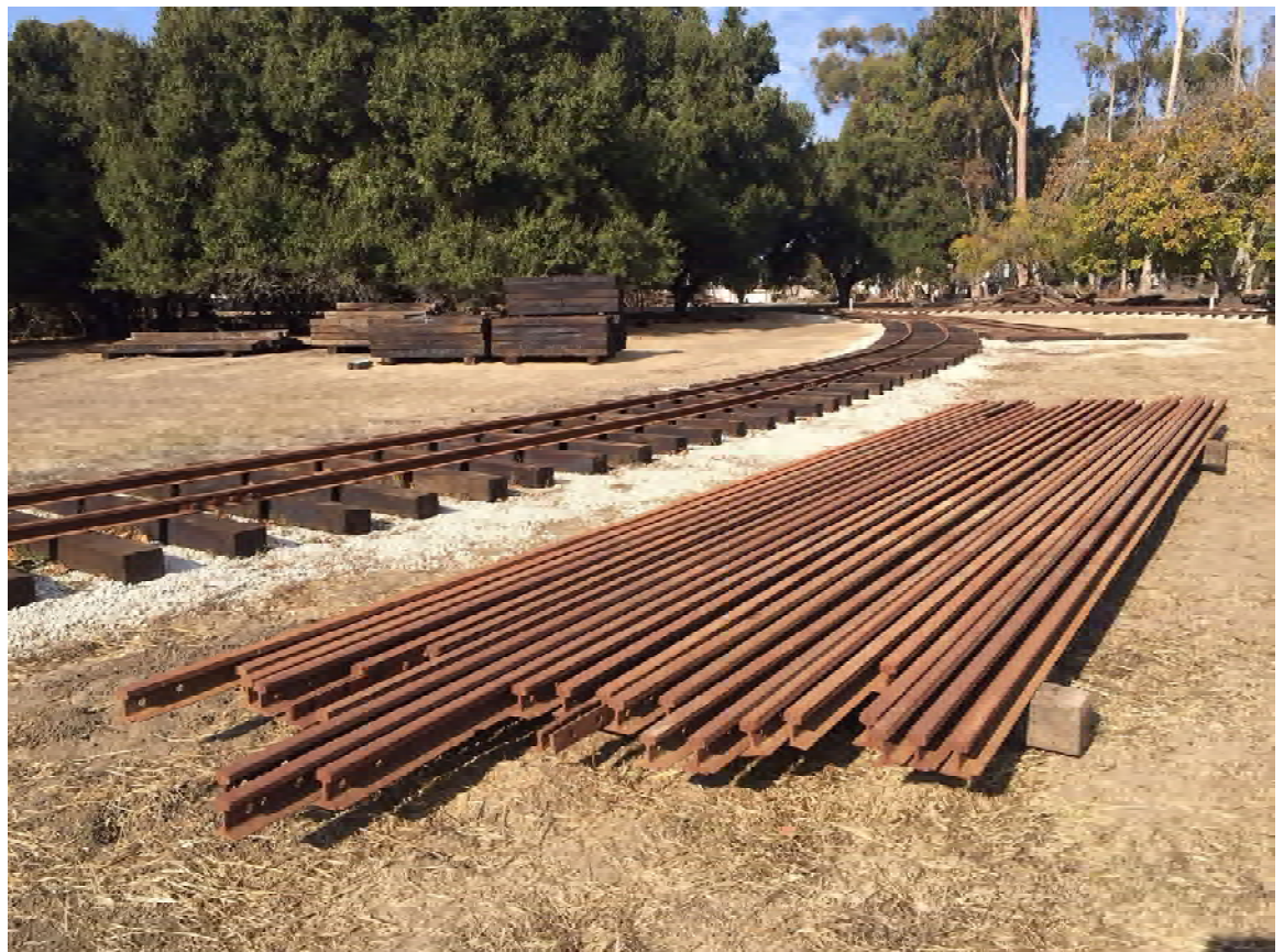
Looking back (east) at the switch shown in the top photo. This track was previously approved in the Car barn phase and was laid in 2020 while we waited for EBRPD approval on mainline extension/loop. The rail in the foreground was acquired years ago from the SF Muni and is 50#. Most of our railroad is 40# rail, so this section of 50# mirrors the original SPCRR that also used 50# rail.
