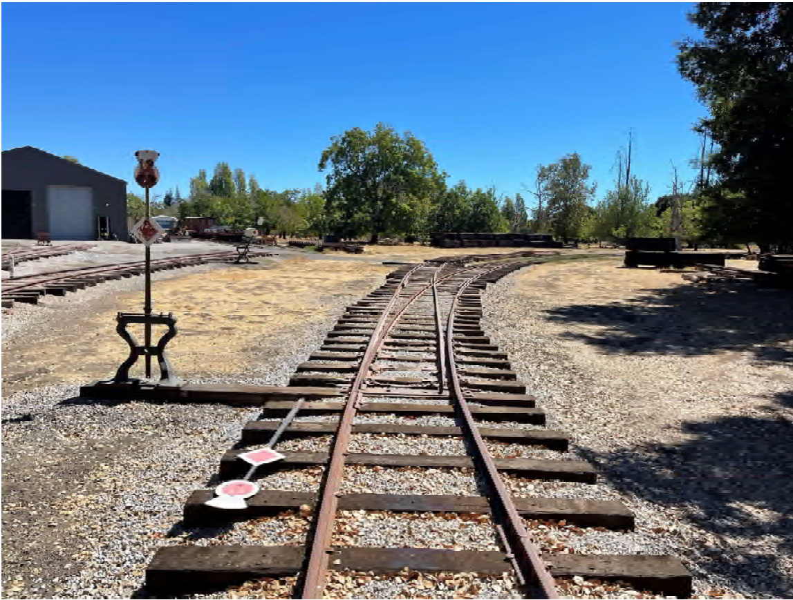
The first switch on the new track for a new storage track (looking west).
