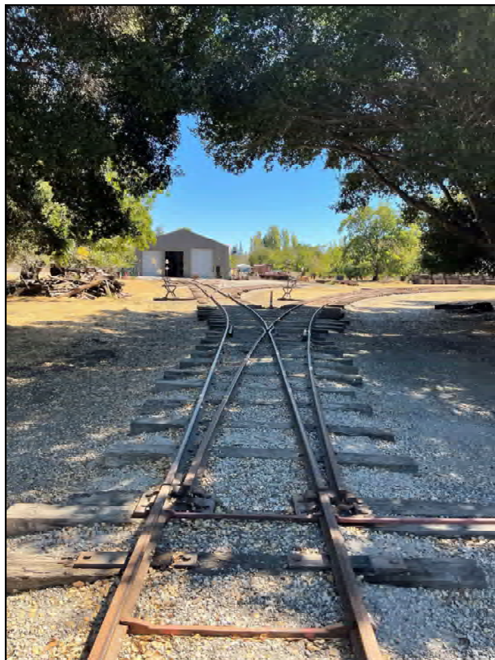
This photo was taken facing south. Shown is the new switch with the new track heading west. Photo: JS Burgess
