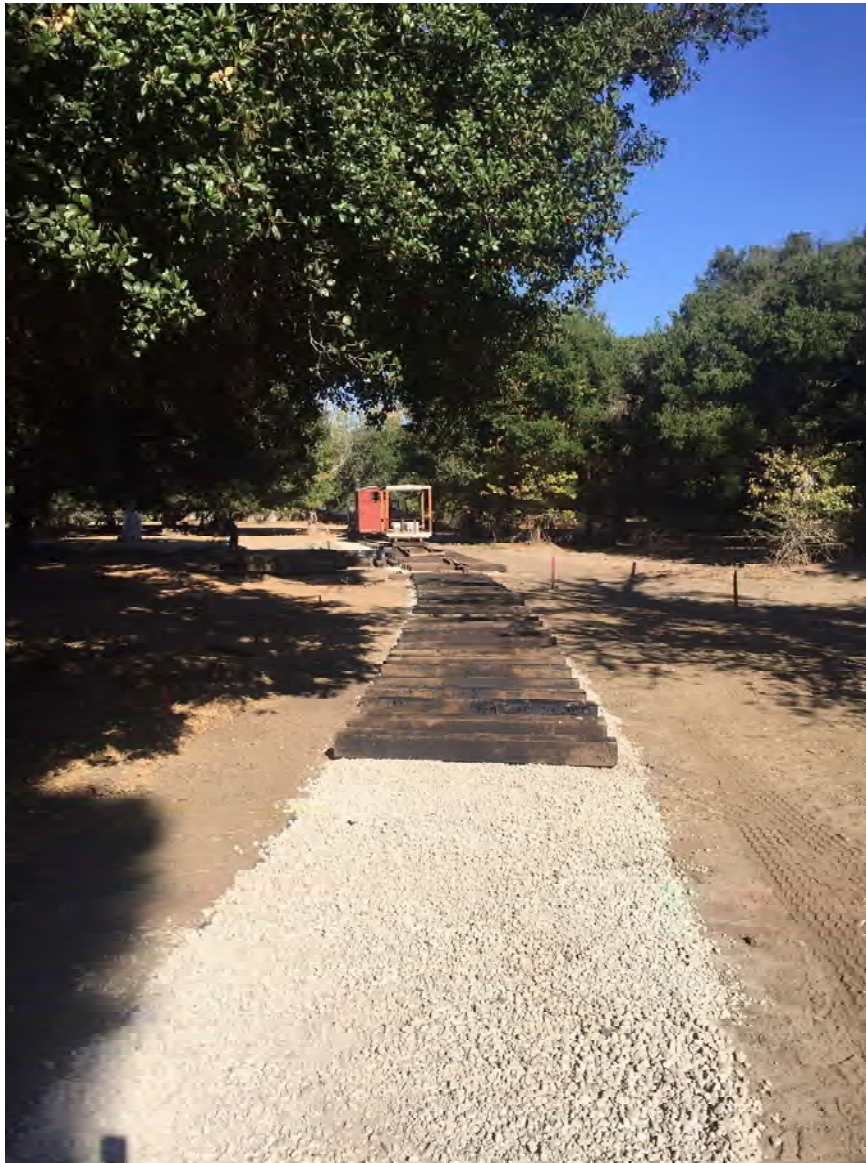
Here we see the next 60 feet of ballasted subbase and ties awaiting rails and spikes. Photo: John Goldie
