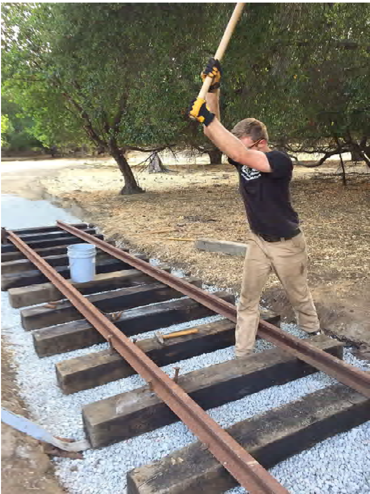
Looking west from the William Patterson road crossing. Bobby Goldie spikes the first section of rail. Photo: John Goldie
