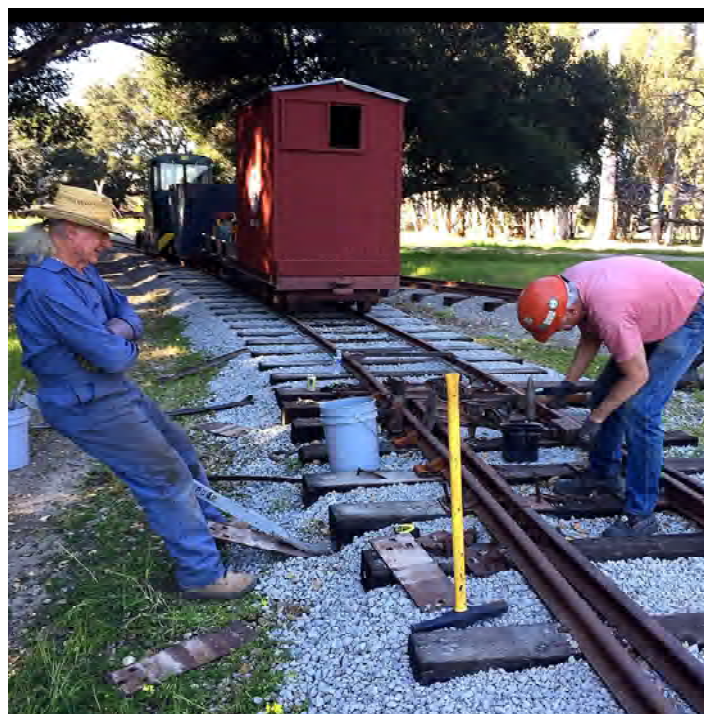
Bruce Sorel sighting down the rail head to check the level of the track. (2/6/22) Bruce and Steve working on the Shop Switch. (2/20/22) Photos – John Goldie
