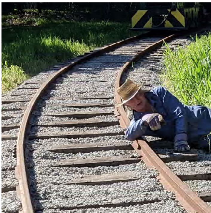
Bruce Sorel sighting down the rail head to check the level of the track. (2/6/22) Bruce and Steve working on the Shop Switch. (2/20/22) Photos – John Goldie
