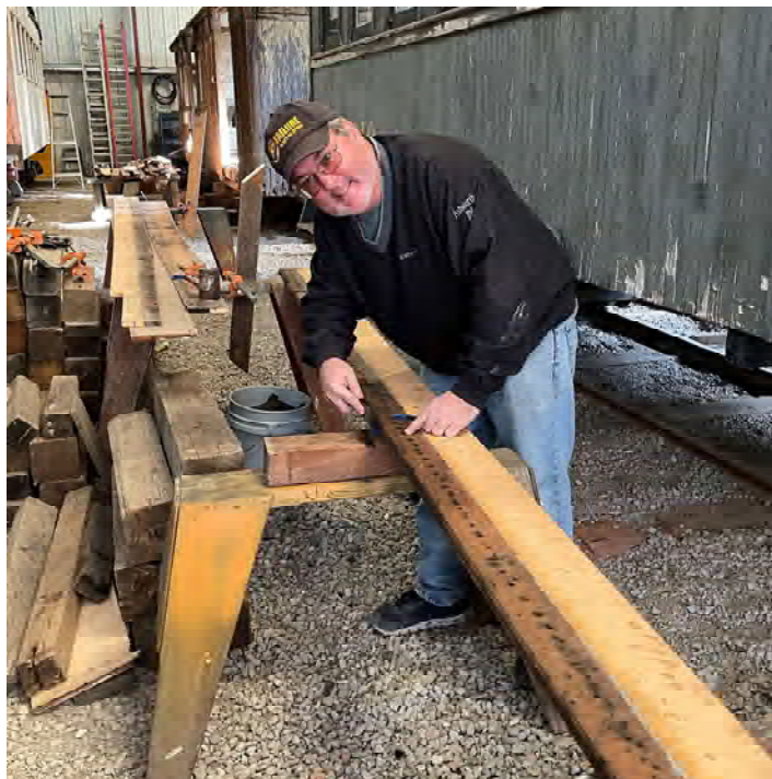
John Erdkamp repairing blemishes and filling tack holes with epoxy resin. (2/21/22)
