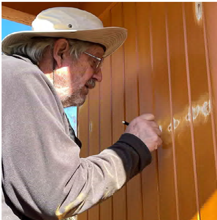
John Stutz meticulously cleaning out caulk that had shrunk using an Exacto knife pointed blade. You can also see the beautiful final color. (2/21/22)
