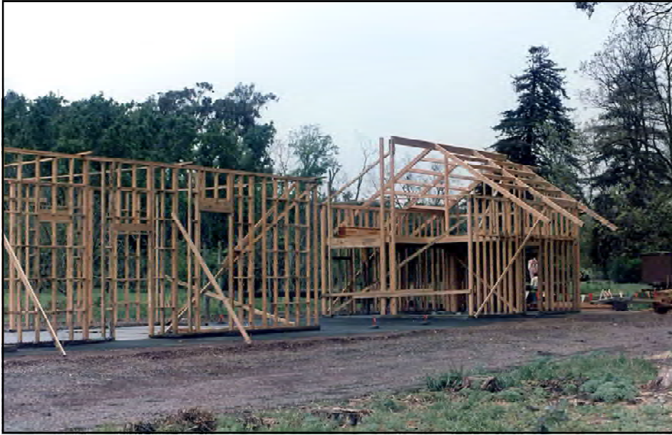
The station and restrooms for the Ardenwood station in 1986. Wall framing is now underway.
