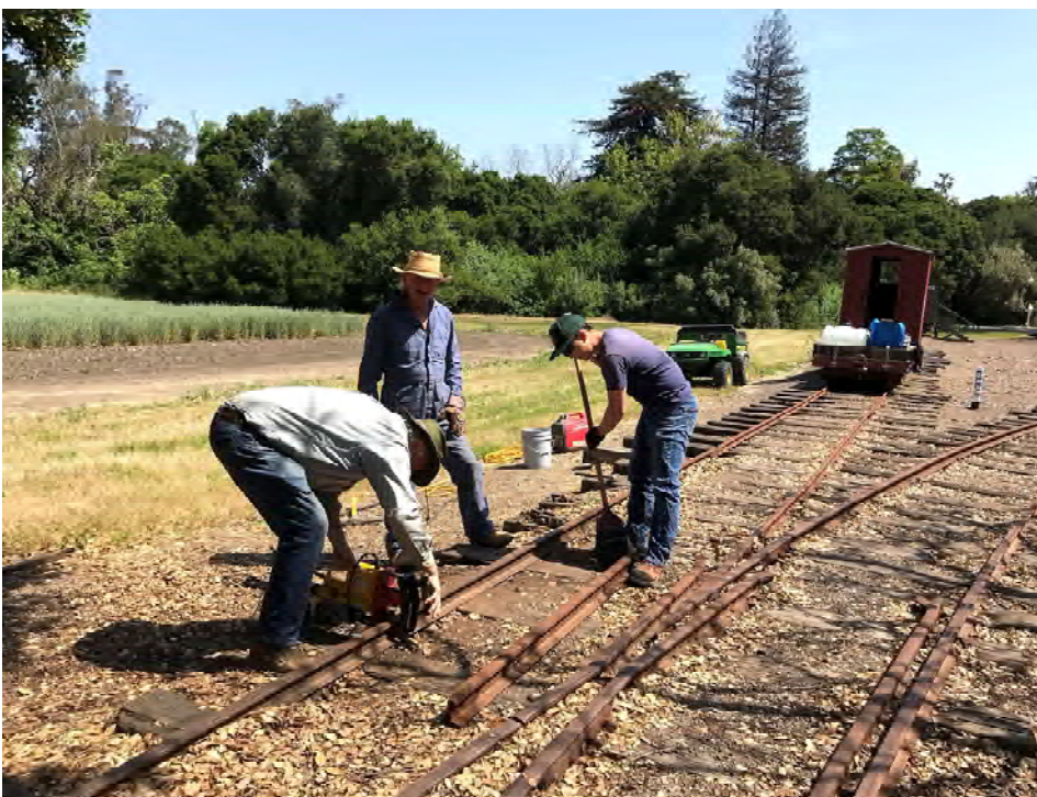
-Track crew working on Shirley's Siding on regular operating day. Photo - James Link
