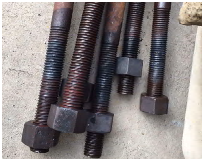
We have 50 rusted track gauge rods. After burning the rust off and cleaning, these are now back in service. Photos - John Goldie
