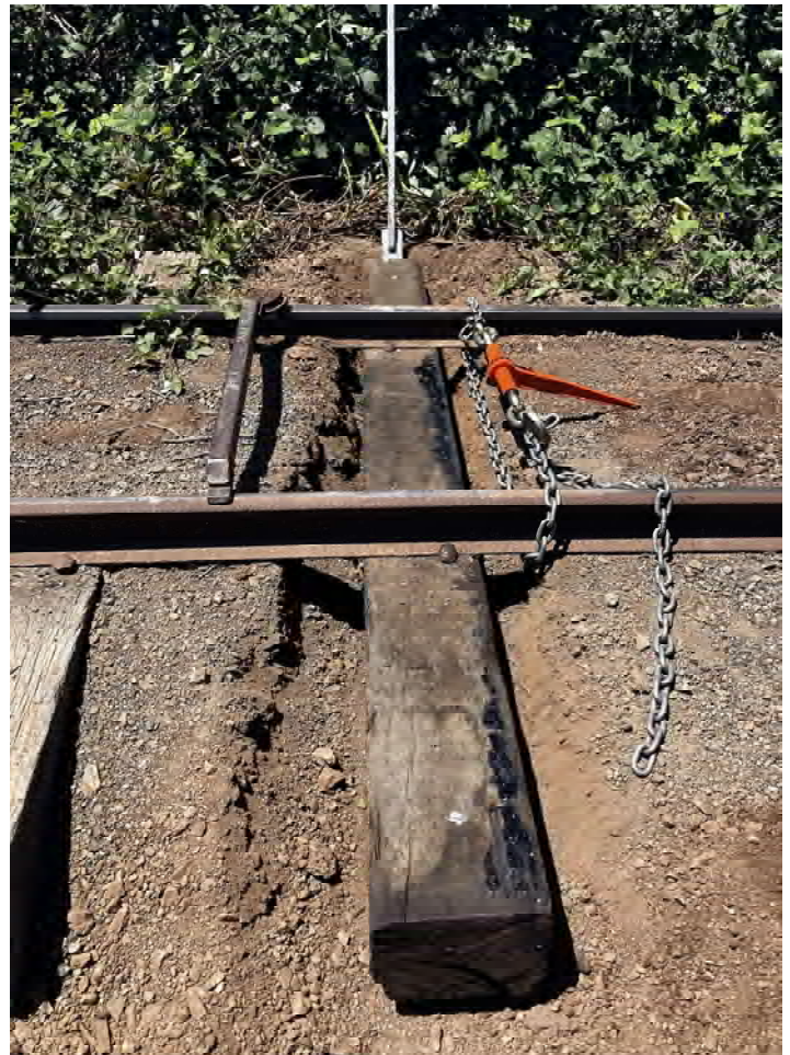
New chain binder being used to insert replacement tie.
