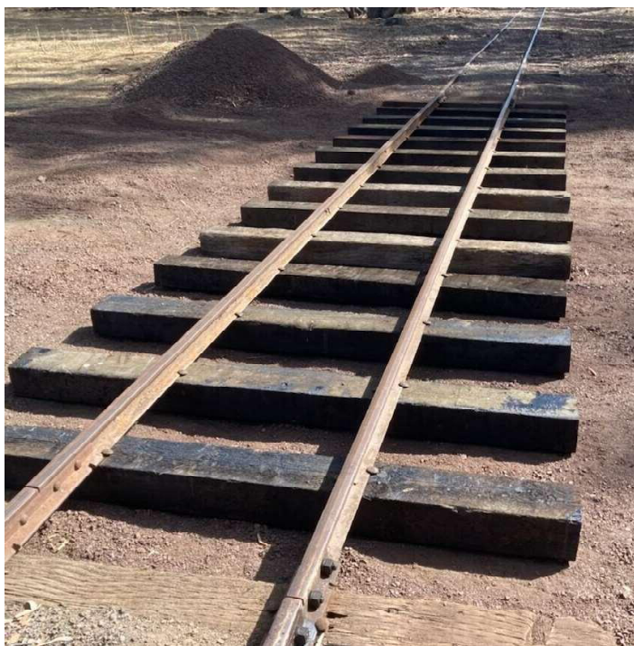
First the rail was removed and the bad ties dug out. Next the new ties we laid out and the rail was replaced.. Photo - David Waterman
