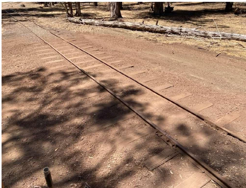
The completed ties replacement.
