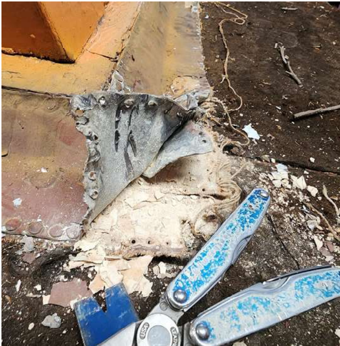
NWP 6101 - Removing lead flashing at base of cupola. Photo -AJL Cary
