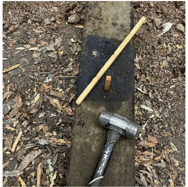
Old spike holes are plugged.
