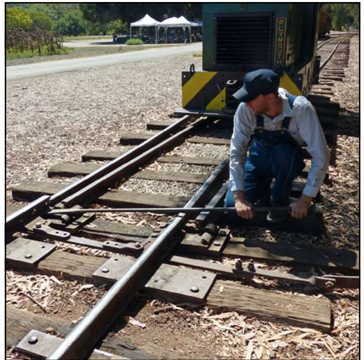
Isaac Sattler tries to pry open the stuck switch.
