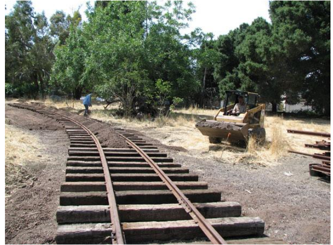
Ballasting the track - photo by AJLCary
