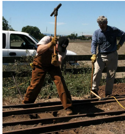
-Spiking Rail at Shirley's Siding Switch - Image AJLCary
