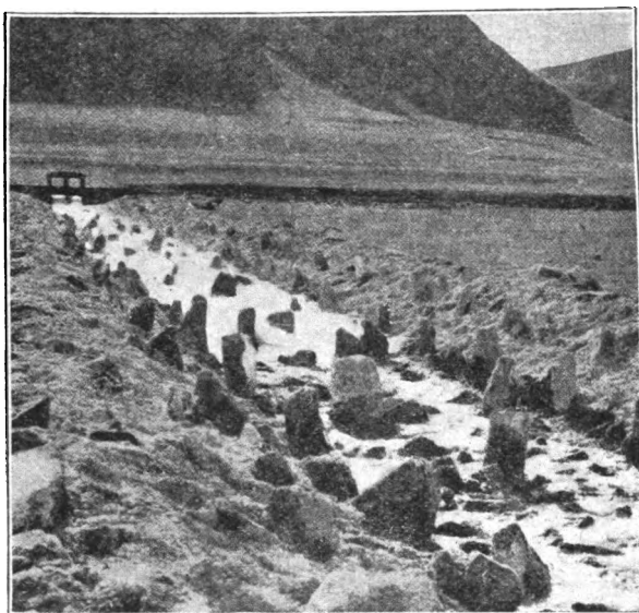
Fig. 26. Chute in Natural Earth; Bed Protected from Erosion by Boulders
