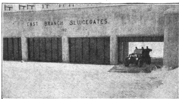
Fig. 117. Typical American Regulating Sluices in Reinforced-Concrete Weir
