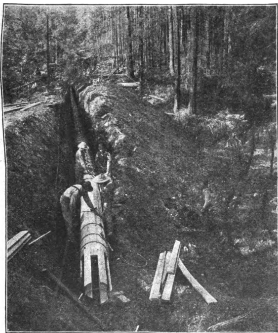
Fig. 30. Erecting a 12-Inch Pipe of California Redwood
